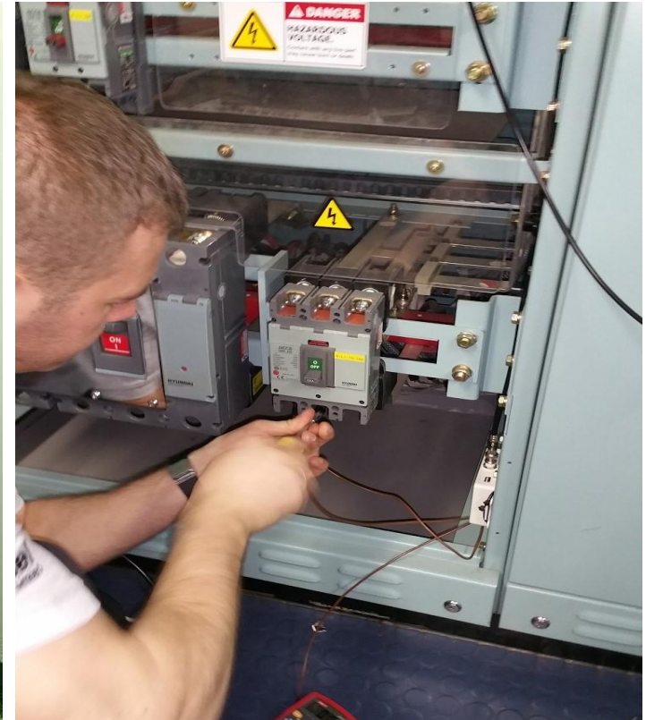
Connecting the 5+1 Coupler onto the Breaker
